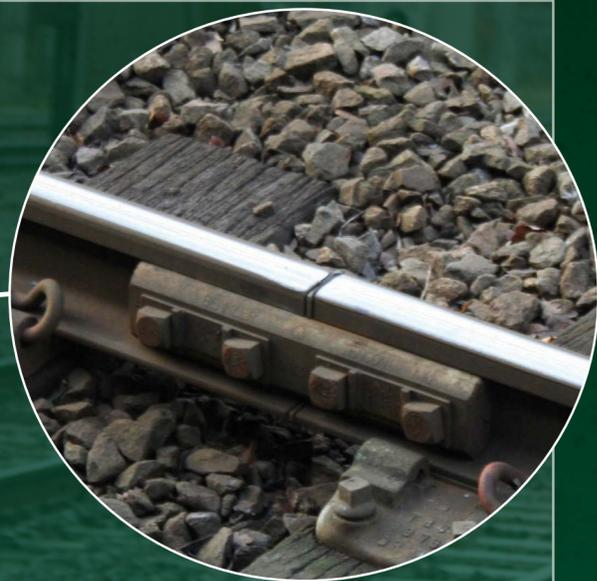
Railway tracks can be made of connecting pieces of rail that are usually 60 feet (18.288 m) long. The pieces are either bolted or welded together at the ends.
